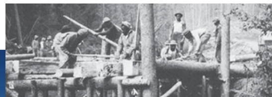
Sikanni Chief River Bridge
